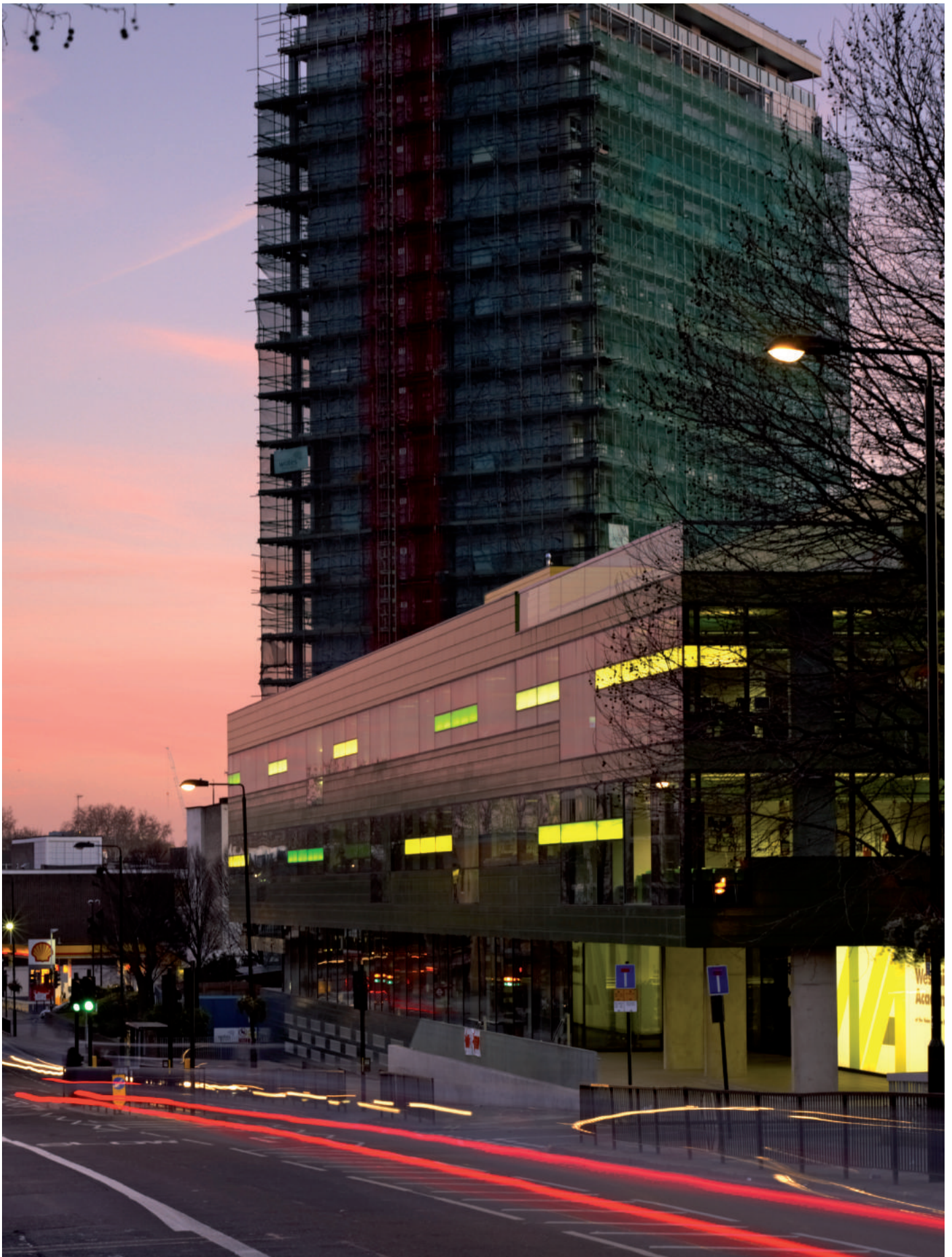
North façade, Harrow Road, at dusk
