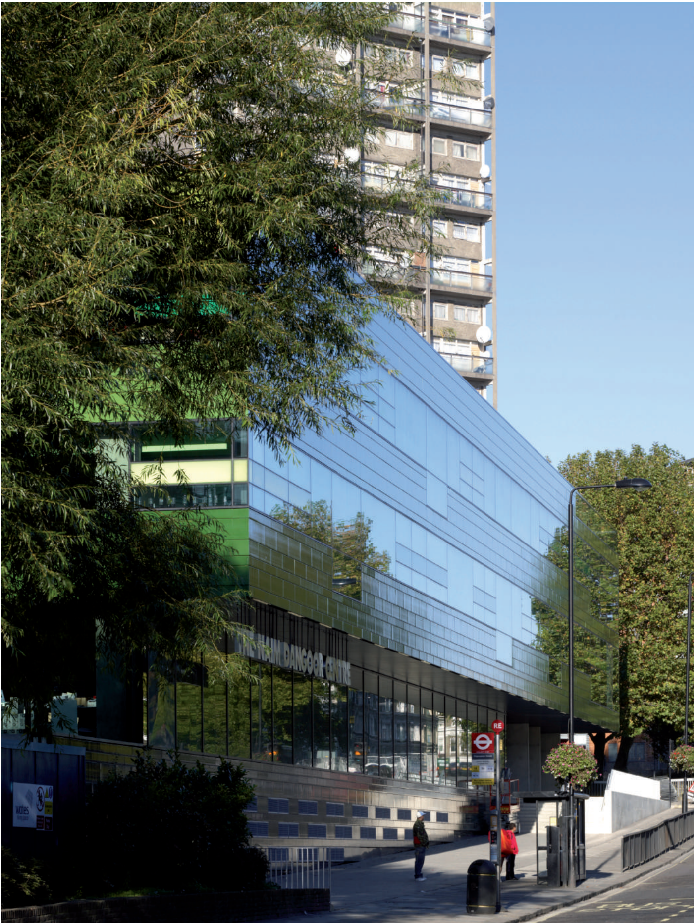
North façade Harrow Road
