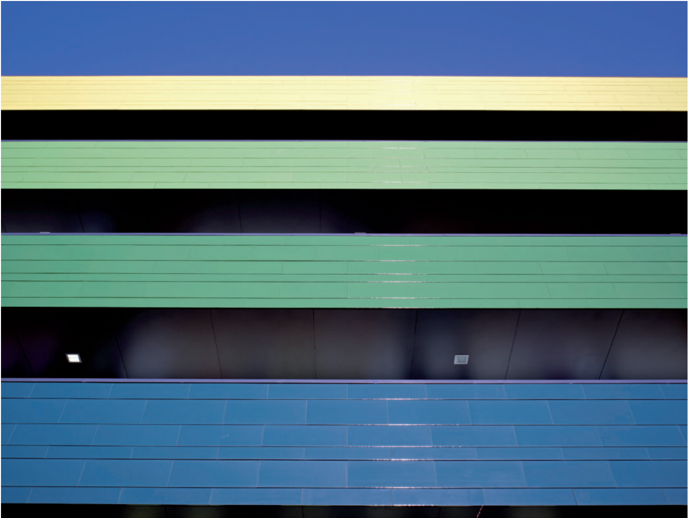
South façade detail
