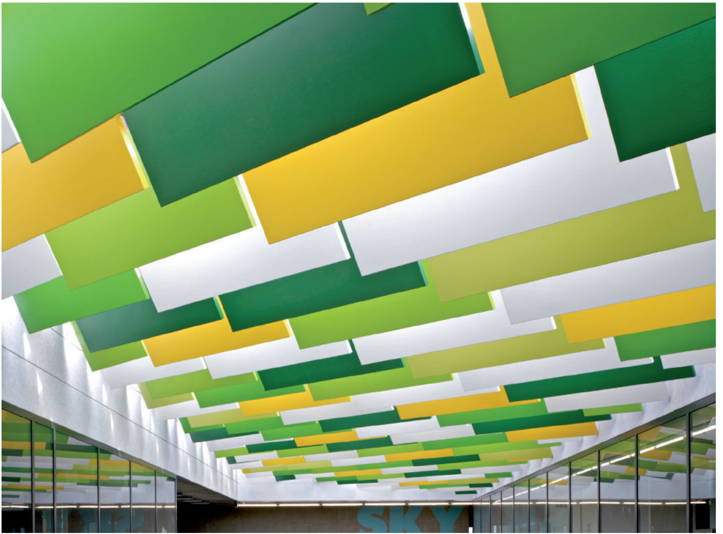
Detail of atrium roof baffles
