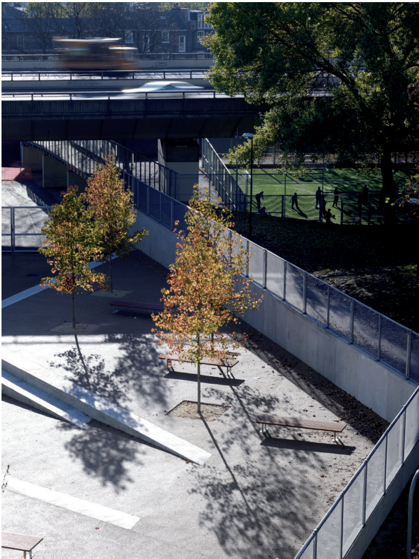
External Terrace spaces and Sports Pitches in the background
