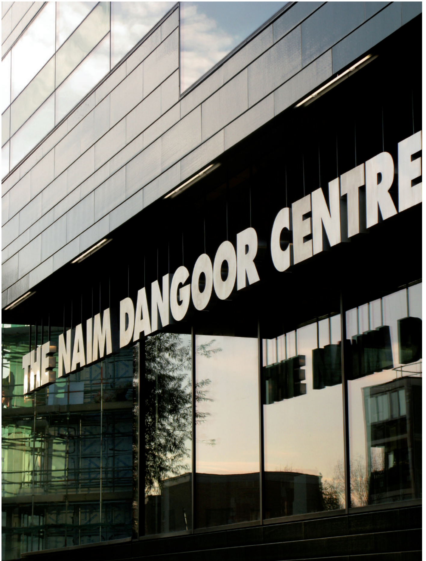
North façade detail
