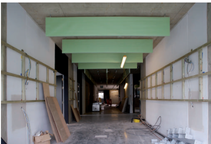
Construction- internal cladding and supergraphic installation
